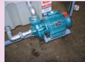
1 hp high pressure & high discharge pump set
